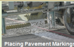
Placing Pavement Markings
